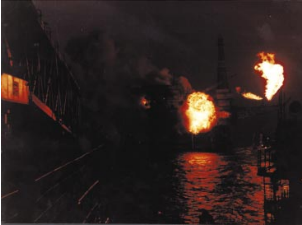
Figure 7. Fireball seen emanating from west face of Module B (cf. figure 2). The HP flare is seen to the right and the fire on the north face is seen to the left. Photograph taken some 15 s after initial explosion.
